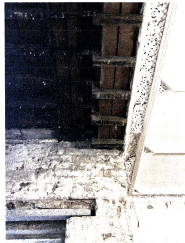
Bay Window Timber beams bearing ends to be checked for rot.
