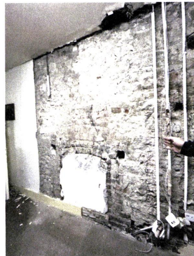
Teacher's Room - Walls treated.
