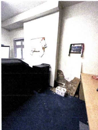
Manager's Room rhs chimney
