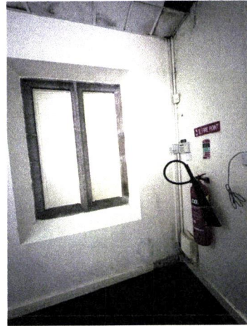
Other side of wall - concealed window.
