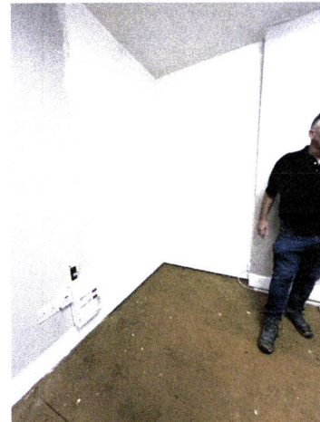
Dean's Room - Diathonite Lime and cork. Photo taken 16-07-2024.
